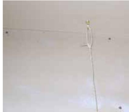
Then a point on the ceiling was selected, and a small hook located there, and a plumb line dropped.
