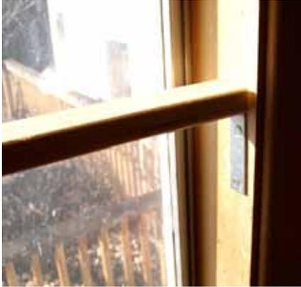
First, a place was estimated about where to place a mirror. Then in this case a cross piece was affixed to both sides of a window frame. This was level in all axes.
