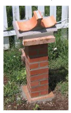
So the column was built up but part way it was time for a cup of tea. After the cup of tea, work resumed however the author mistakenly didn't alternate one layer of bricks.
