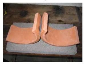
The two semicircles are tacked together with an epoxy and allowed to set overnight. Later the upper space between the curved dial plates as well as the lower space adjacent to the mounting paver will be filled with mortar.
