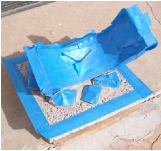
The dial protected with masking tape before mortar was applied. Mortar was used rather than sanded grout, this was to generate a coarser finish.
